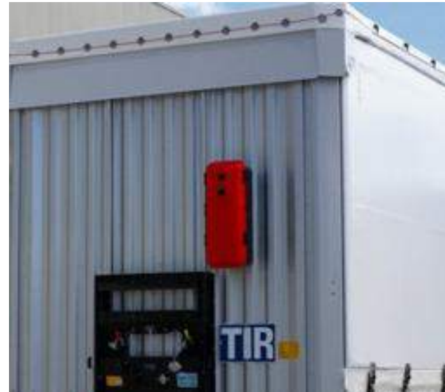
1 unit of fire extinguisher box on the front panel
